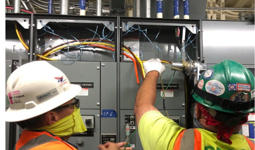
New Motor Control Center Installation
